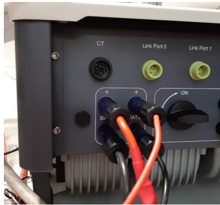
Figure 60 - Inverter-side DC power connection with two battery inputs populated
