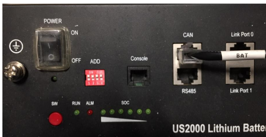
Figure 12 - Connecting the communication cable to the Pylontech battery
