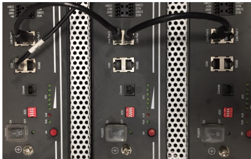
Figure 14 - Connecting the communication cable between three Pylontech batteries
