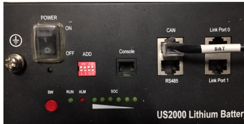
Figure 9 - Connecting the communication cable to the Pylontech battery
