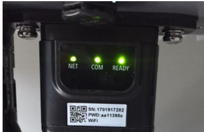
Figure 103 - Final status of LEDs
