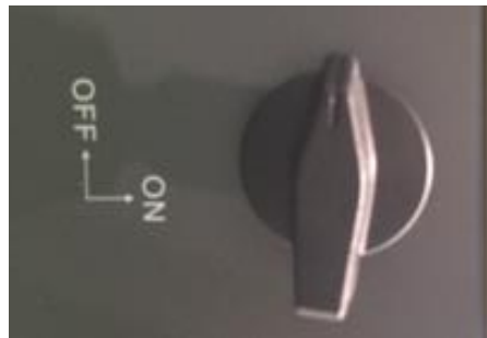
Figure 67 - Photovoltaic disconnecting switch
