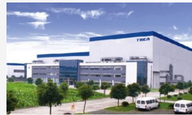
Shanghai EHV Electrical Science and Technology Industrial Park (Shanghai)
