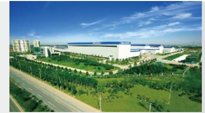
The Northeast Industrial Park (Liaoning)
