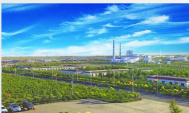
Zhudong Coal Power Energy Base
