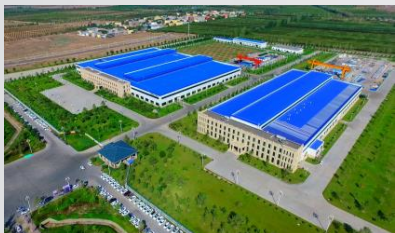
TBEA Intelligent Electrical Industrial Park
