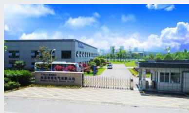
Nanjing Intelligent Electrical Industrial Park (Jiangsu)
