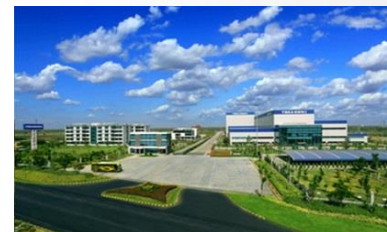
India 765kV EHV Power T&D Hi-tech Industrial Park
