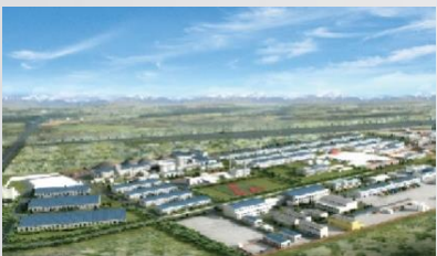
Joinworld New Material Industrial Park
